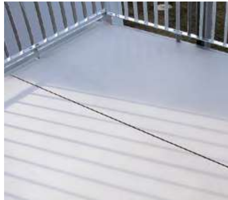
INCLINE AND PANEL JOINTS
