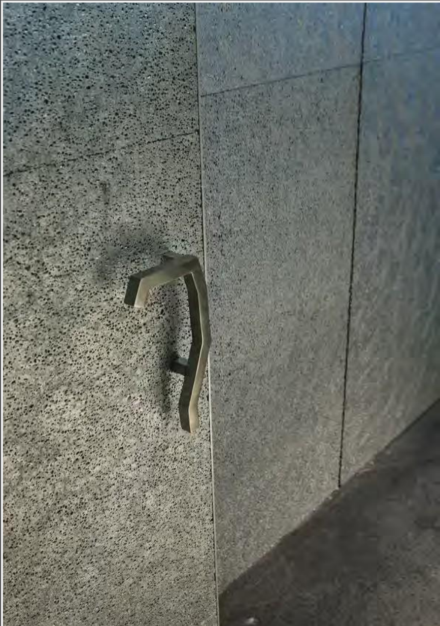
Vanke Centre, China – Steven Holl Architects ALUSION™ Wall Cladding, in a Geometric Configuration ALFG-12.7-SM-1S, Small- Cell Open on One Side, (Top side), Thickness: 12.7 mm (0.5")
